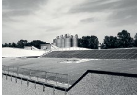
4'173 photovoltaic panels on the rooftop of the Artigo plant
