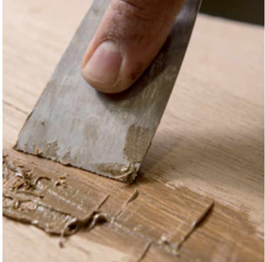
Filling of the knots and cracks
