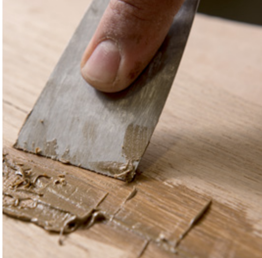
Filling of the knots and cracks
