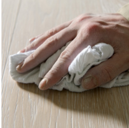
The technique of applying colour by hand with rags
