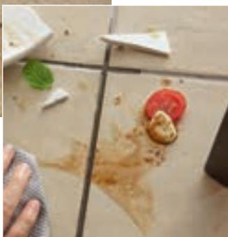
Cement joints between tiles soak up liquids and oils and are often permanently discoloured.
